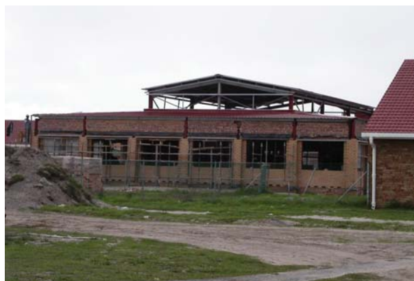
This is the new Indoor Hydrotherapy and Gymnasium building.
